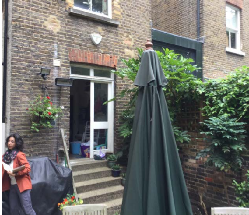
View of location of two storey rear extension to the closet wing at lower ground and ground floor levels.
